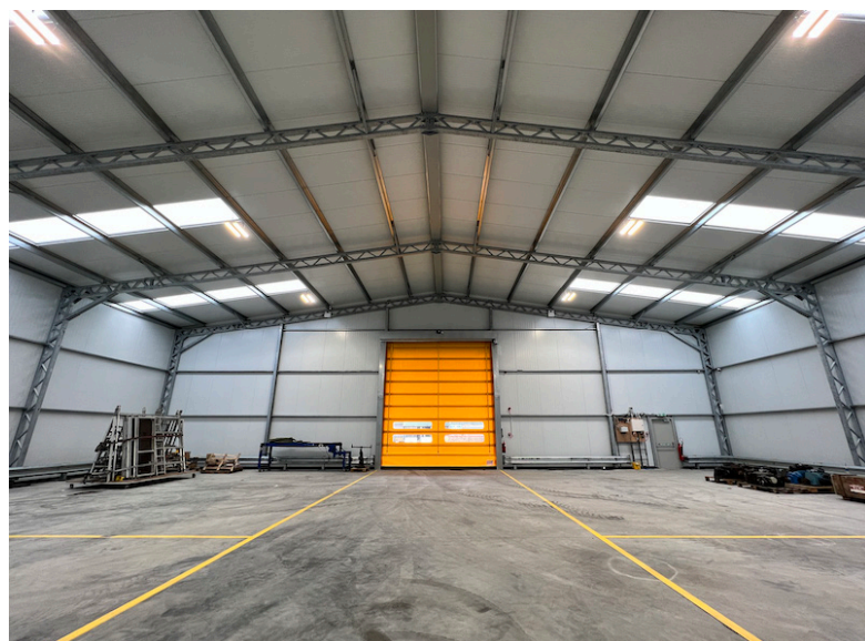
INSIDE THE MAXI-SPACE STORAGE FACILITY WITH COMPOSITE ROOF
