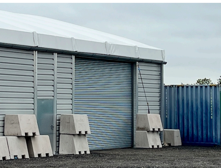
RELOCATABLE CONCRETE BLOCKS USED TO WEIGHT THE BUILDING
